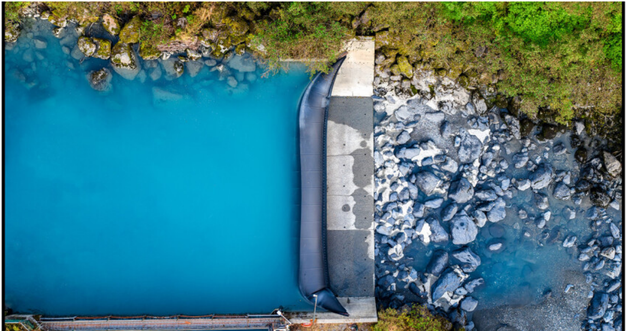
Power Creek dam in Cordova, Alaska, provides 65-70% of the community's electric power. Photo by Seed Media for Cordova Electric Cooperative.
